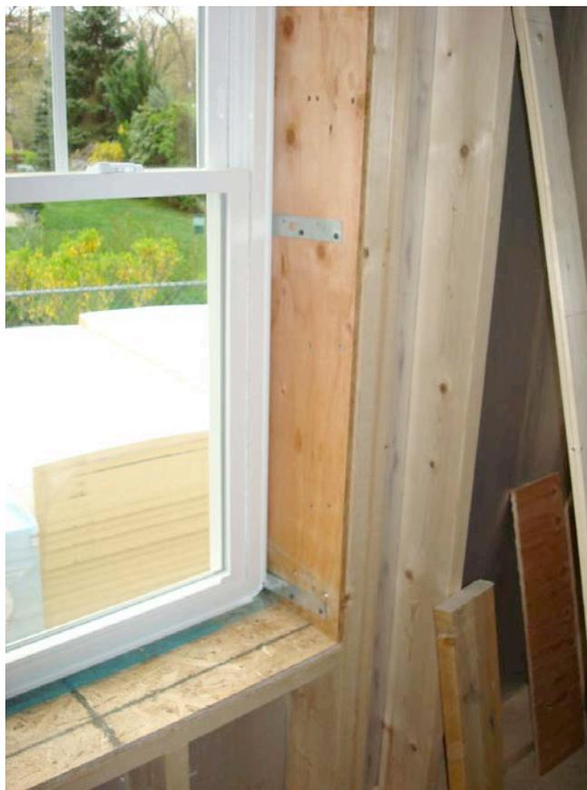
**Photograph 3: Strap Window Attachment**—Similar to window installation in masonry opens lined with window bucks. Unlike masonry openings the window flanges are retained for water control.
