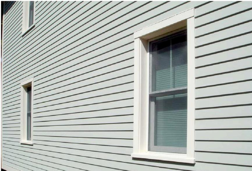
**Photograph 1: Beautiful “Innies”**— The trim is returned to the flange or face of the inset window. The flashing at the top of the window opening at the horizontal strip of head trim just covers the top of the trim itself—it only protects the top of the trim - it does not have to extend to the back of the continuous insulation and connect to the face of the structural sheathing/water control and air control layer.
