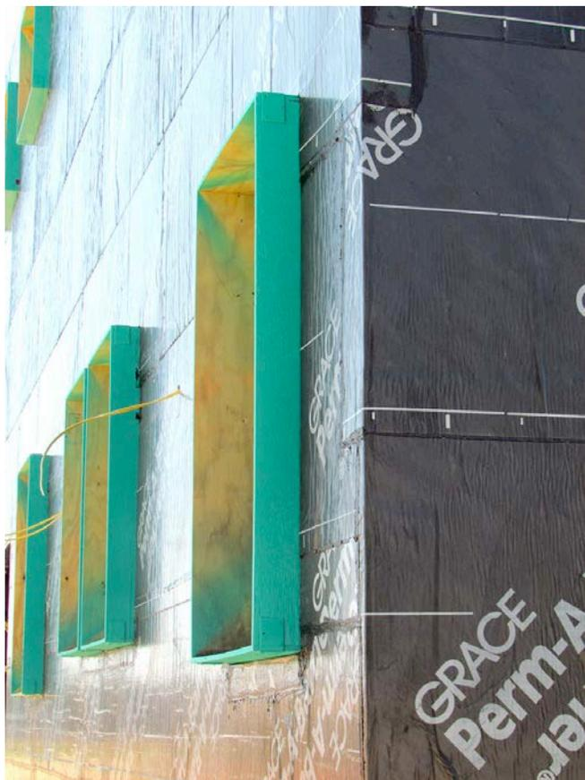
**Photograph 2: Structural Box**—Typically plywood or OSB protruding past the exterior face of the framing extending the thickness of the continuous insulation. How thick can you go with the continuous insulation with the structural box? Typically 4 to 6 inches.
